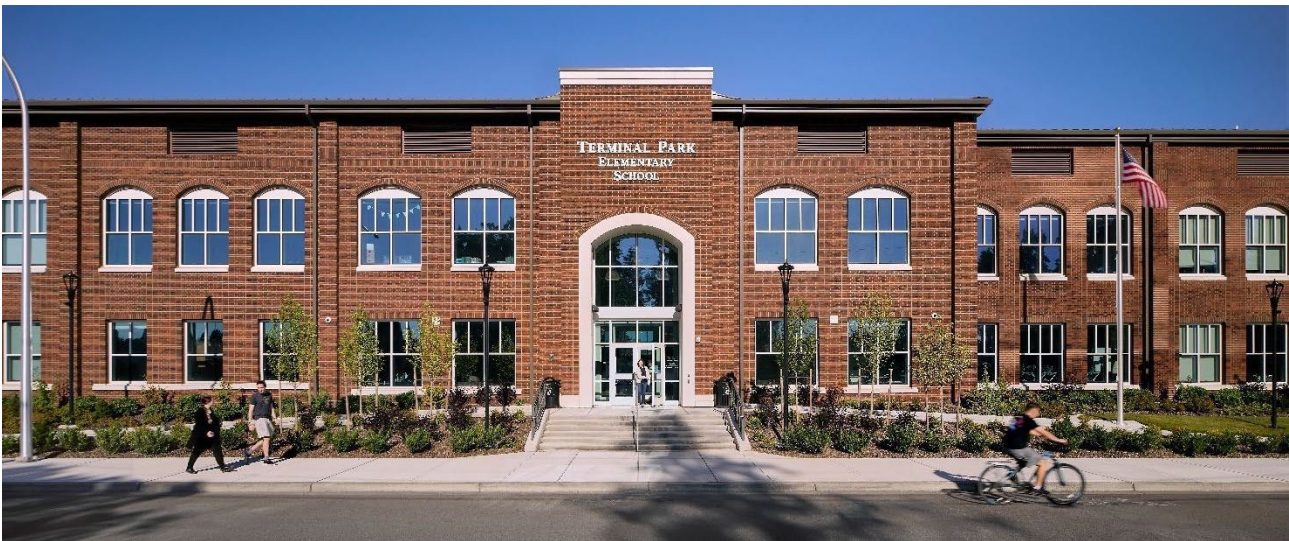
Terminal Park Elementary School – 2023
