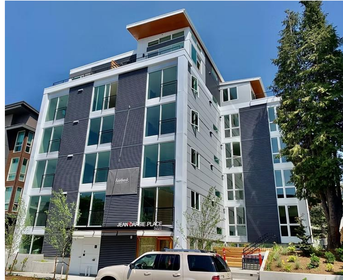
Jean Darsie Place, a ROW-funded Permanent Supportive Housing (PSH) building in the U District.
