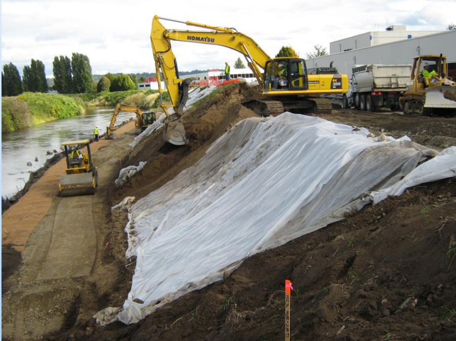
Green River levee construction, September 2007
