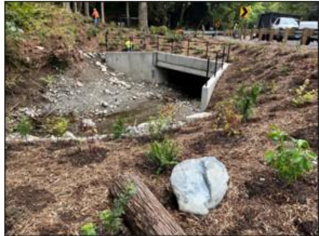
Culvert replacement, NE Woodinville-Duval Road August 21, 2024
