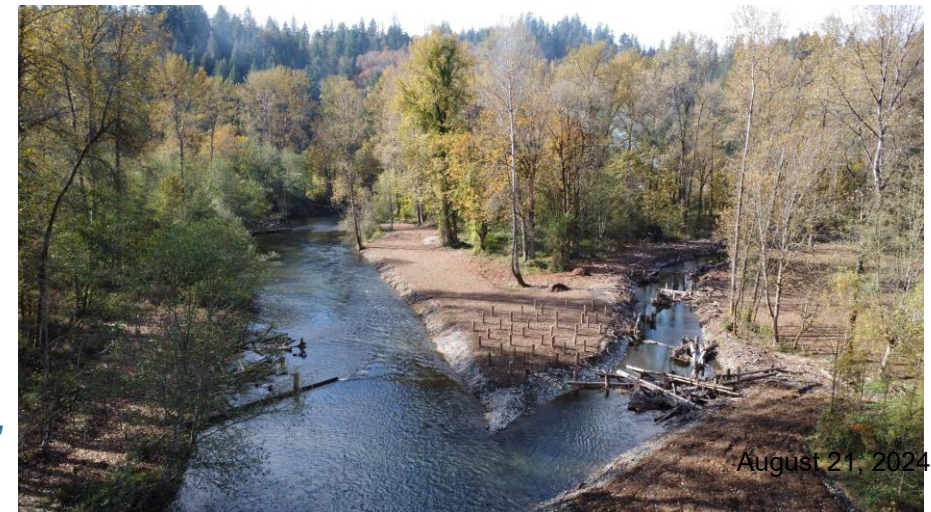
Jan Road Levee Setback, Cedar River, 2023
