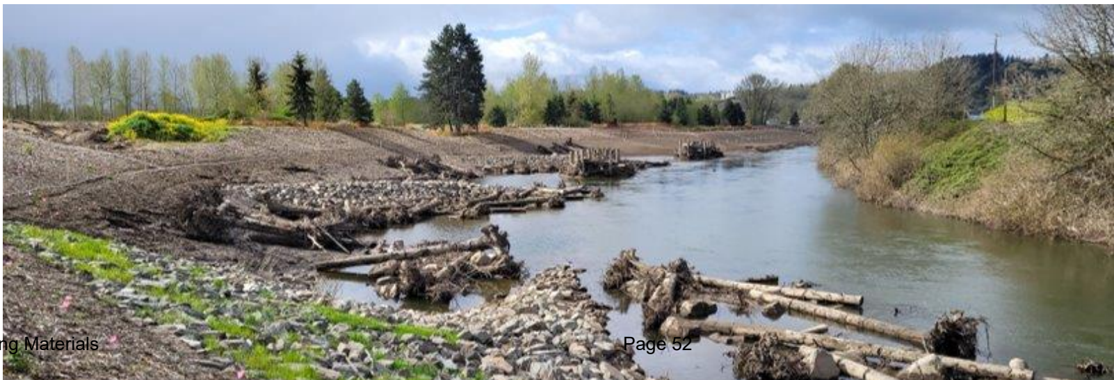
Lower Russell Levee Setback, Green River, 2022
