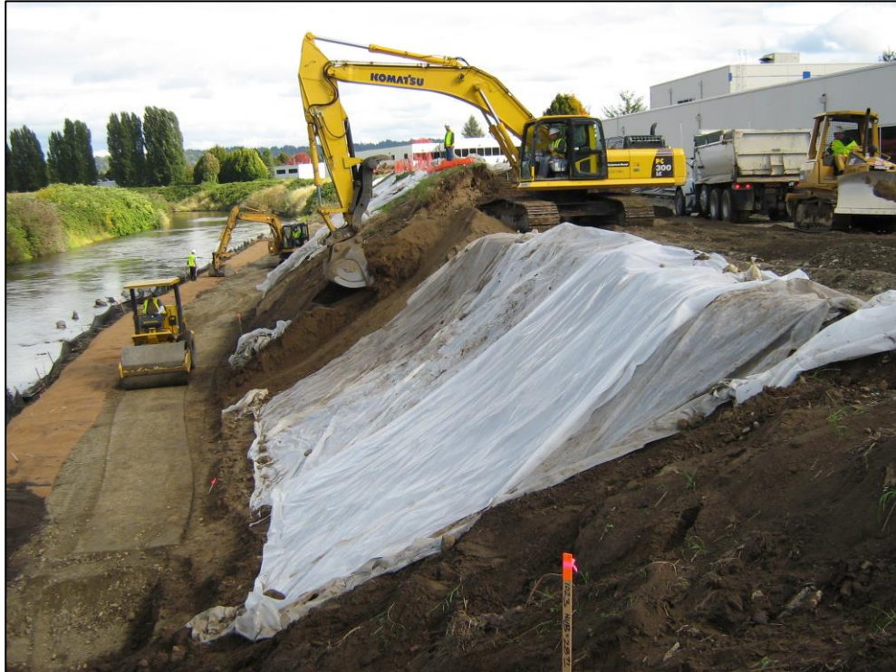
Levee construction along Green River, Sept. 2007
