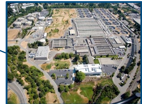
South Plant Treatment Plant
