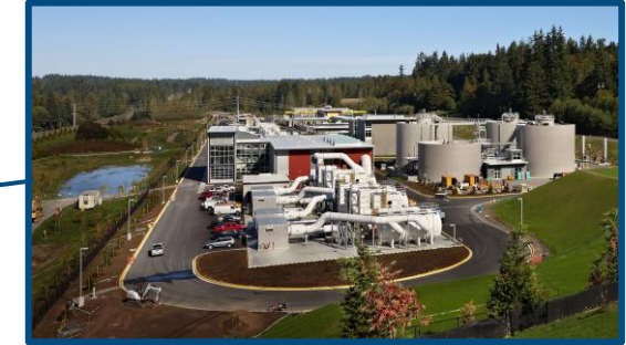
Brightwater Treatment Plant
