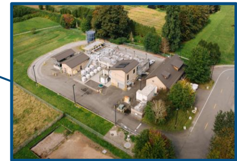
Carnation Treatment Plant
