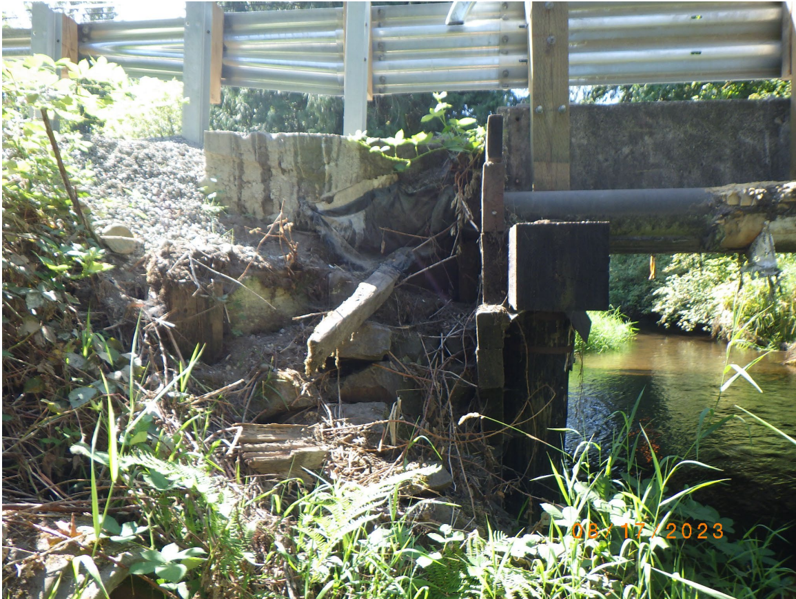
Bear Creek Bridge (9333A) wingwall planks are rotten and failing.
