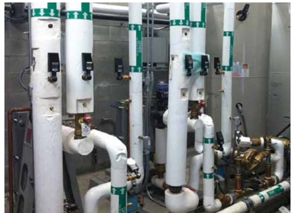
New energy efficient heat exchanger, water piping and controls at the Maleng Regional Justice Center (MRJC)
