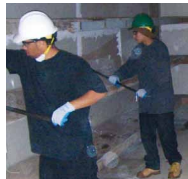
YouthSource crew removing drywall as part of a residential deconstruction project.
