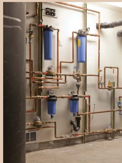
Eastside Harvest House includes permitted potable rain water system - the first in King County
