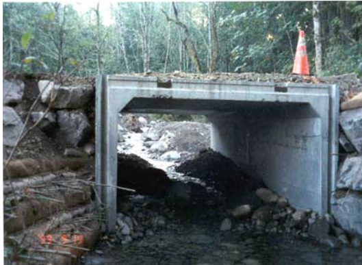
Photos 3 and 4. New box culvert and downstream reach immediately following construction in September 1999.
