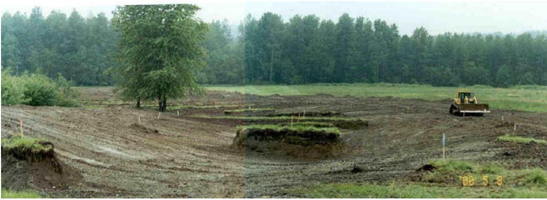
Photo 5. Shaping a broad floodplain bench for the new O'Grady Creek stream channel. May 2000.
