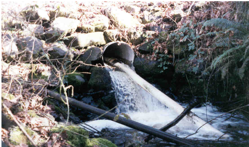
Photo 1. Fish-impassable culvert on O'Grady Creek. Spring 1999.
