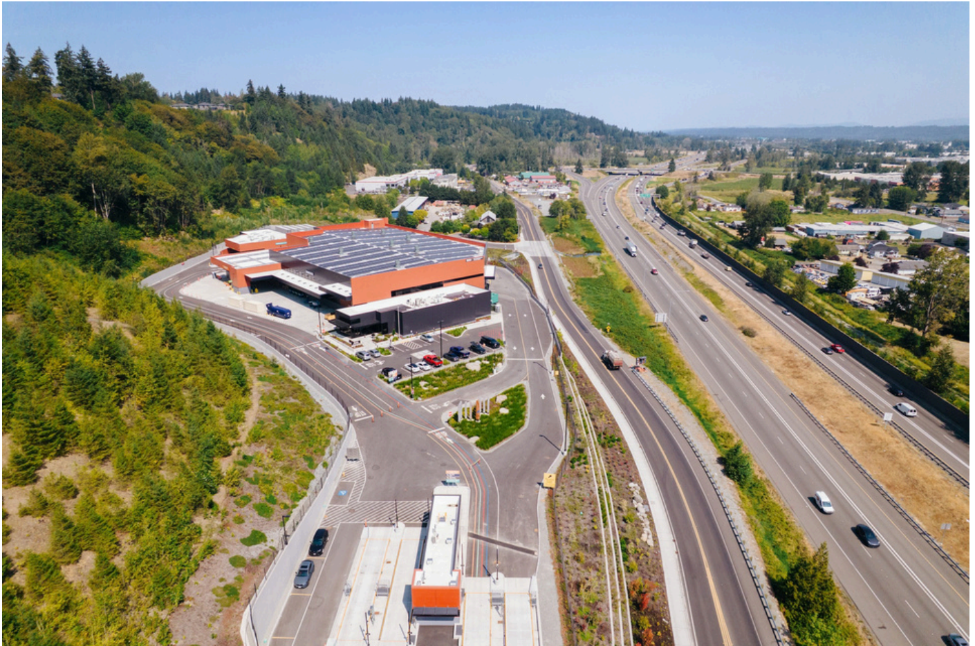
An aerial image of the new South County Recycling and Transfer Station, located on West Valley Highway, west of SR 167.
